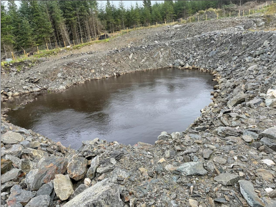
Plate 4--14 Unfilled section of peat cell with artificial pond
