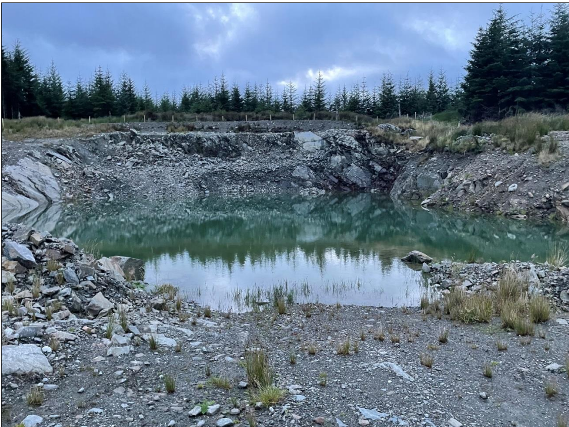
Plate 4-15 excavated peat cell at Deviation 15
