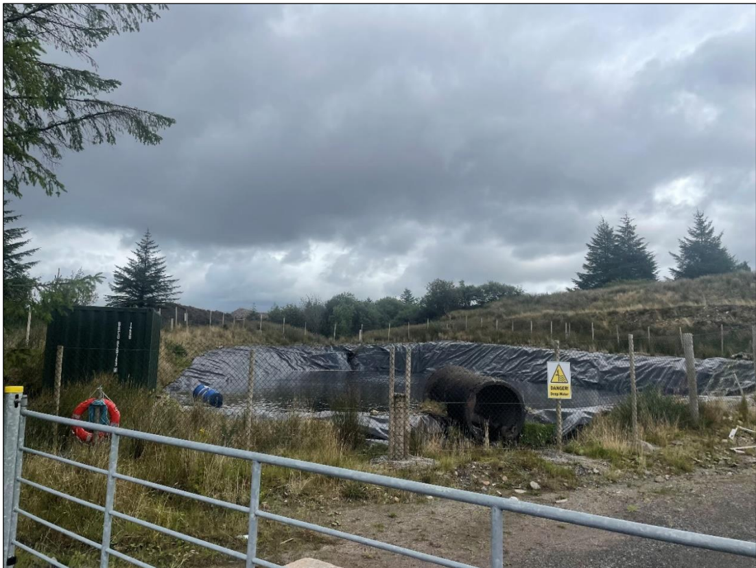
Plate 4--2 Relocated and plastic lined settlement pond showing overflow pipe (August 2023).
