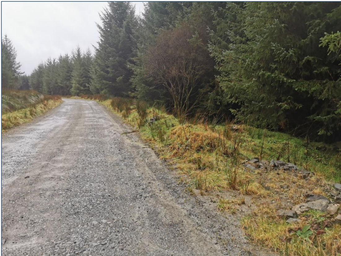
Plate 4--21 Revegetated roadside berm, December 2023.
