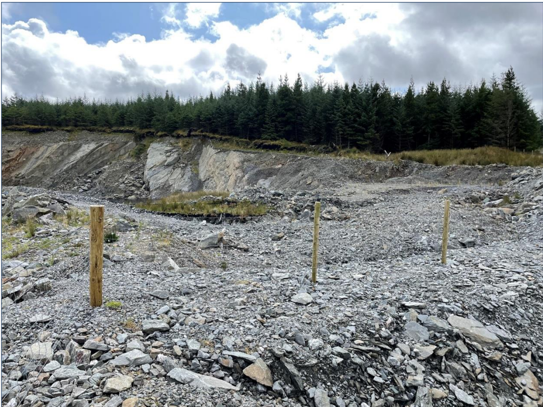
Plate 4--8 Unfilled section of peat cell and conifer plantation on shallow peats in the surrounding area.
