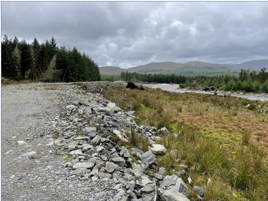
Plate 4--10 Containment berm on left of plate, with amended road to the right. Recolonising habitats visible where conifer forestry has been felled
